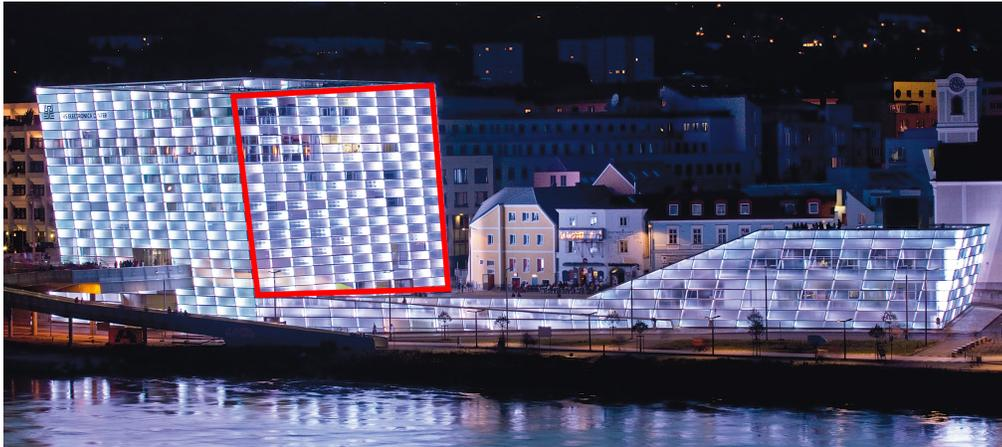
Figure 4.1: The low-resolution media facade of the ARS Electronica Center in Linz, Austria (Photo: Lois Lammerhuber/Photoagentur Lammerhuber). The surface of the building is equipped with about 40,000 illuminating diodes (red, green, blue), turning the windows into pixels. The framed area (red) providing approximately 230 pixels (10x23) was used for the interaction.
