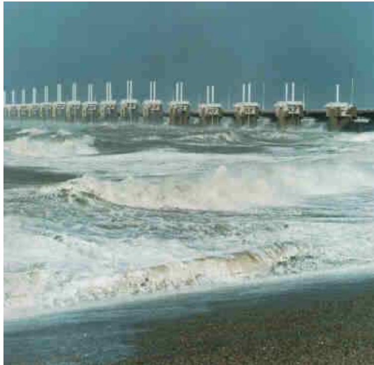
Figure 4.15: The gates of the ECS
