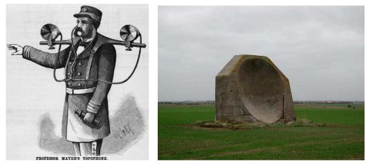
(a) The topophone was an acous- (b) Acoustic mirror near Kilnsea, UK (source: tic based tool for direction es- http://www.geograph.org.uk/photo/315865) timation in maritime applications
