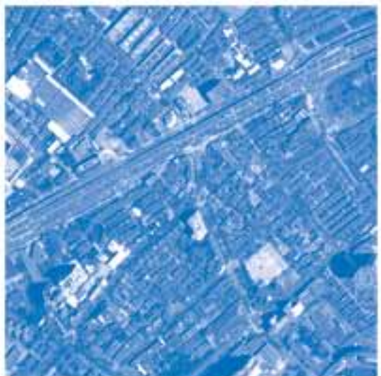
2002 factory district, Shanghai
